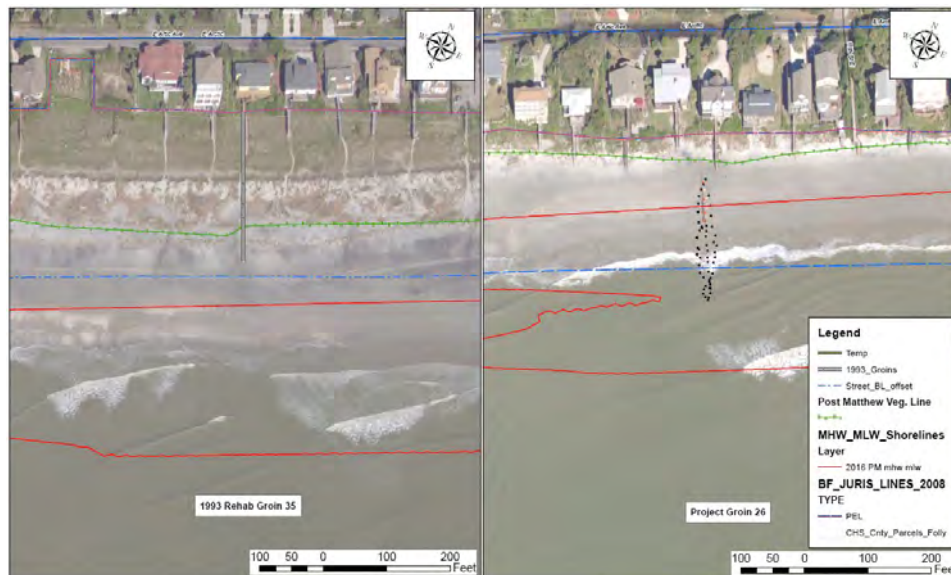
Figure 5. Comparison of beach health at functional (left) and poorly functional (right) groin systems. Note much healthier and wider dune system on the left image.
